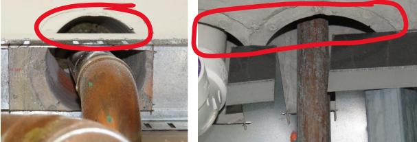
The hole is extending over the fire rated wall stud thickness.
